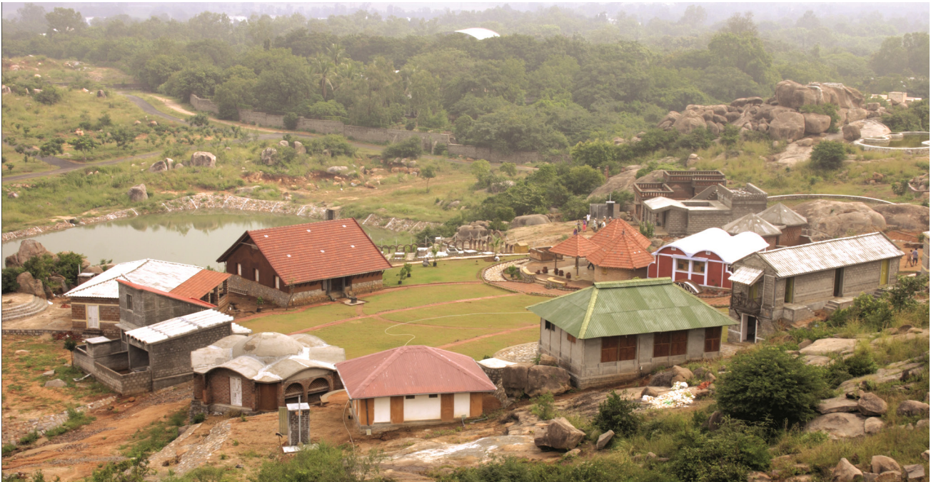
An aerial view of RTP, NIRDPR
