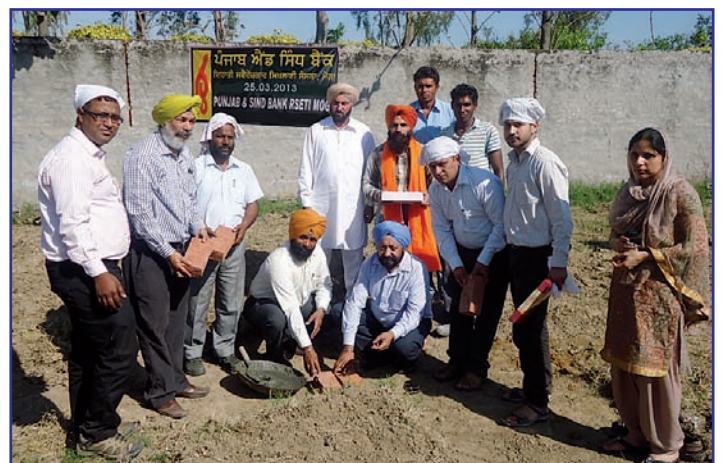
Foundation laying ceremony of PSB RSETI, Moga
