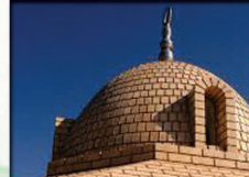
BRICK DOME ROOF
