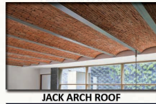
JACK ARCH ROOF
