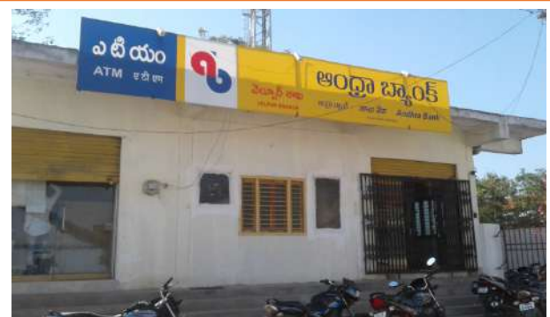
Photo 4: Commercial building rented to Andhra Bank in Velpur GP
