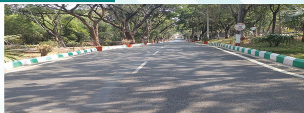
NIRDPR Campus Road laid using waste plastic
