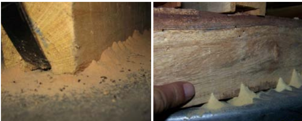
Damage caused by Wood Borer/ Powder Post Beetles
