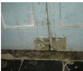
Removing gaps on door joints
