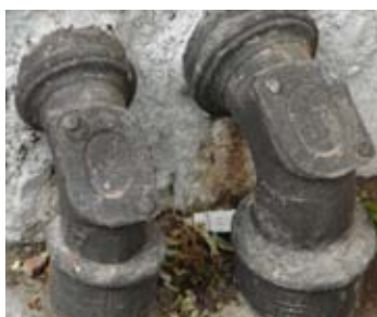
Proper closure of gutter pipes
