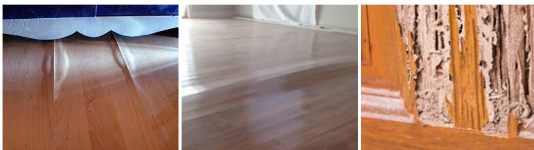
Bubbling or blistering of wood and portion after removal of the surface veneer
