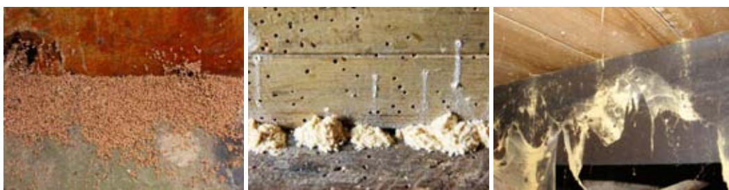
Dry Wood Termite Wood Borer damage Wood borer damage
