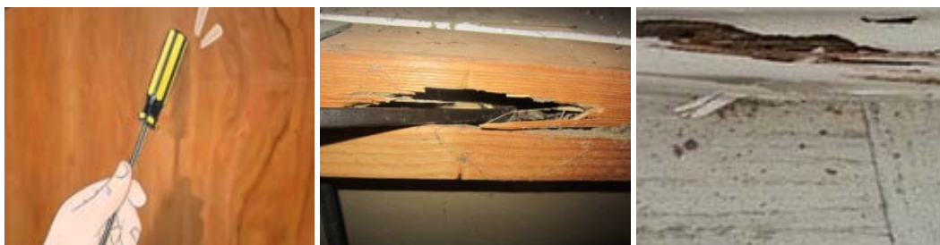
Check the wood for hollowness Pry open Expose the damage
