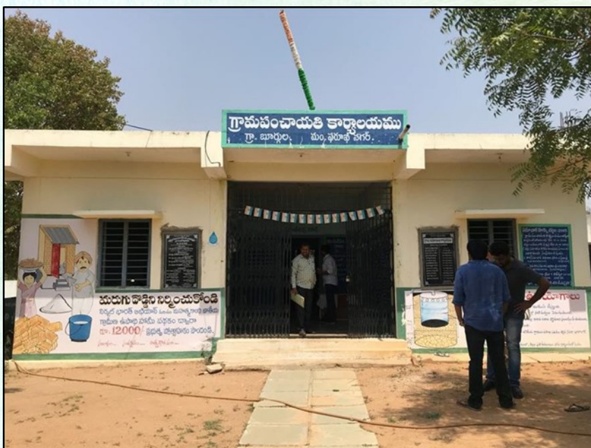
Figure 2: Panchayat Bhavan at Burgula
