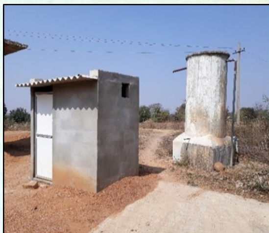
Figure 20: A Toilet Constructed under MGNREGS at Raikal Tanda
