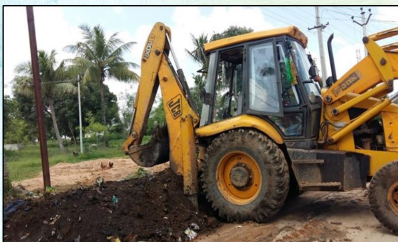
Figure 19: Clearing of Waste Dumped Using Excavator in Progress in Burgula
