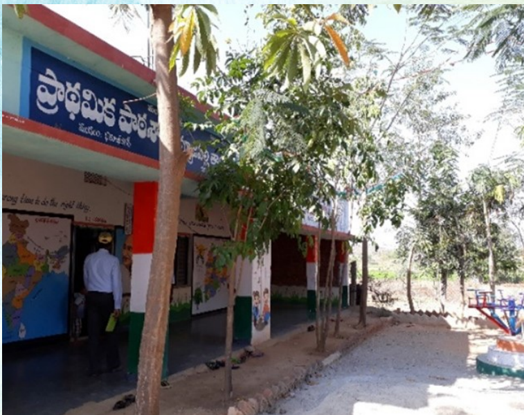
Figure 14: Primary School at Thimmajipalle Tanda
