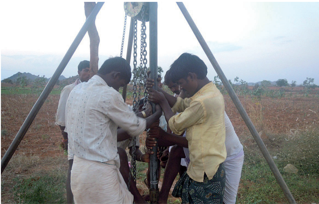
Mallappa and others taking out submersible pump
