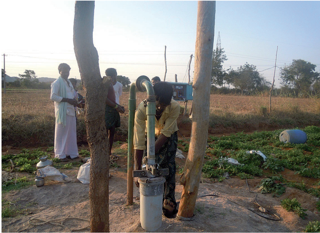
Mallapa and others inserting in submersible pump
